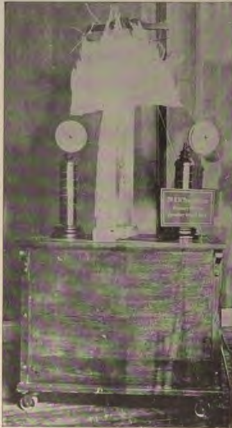
Transformer Discharging Through a 32-in. Gap.
